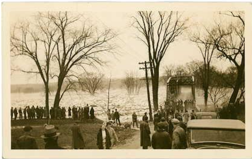
Ice jam and debris- Boscawen-Canterbury Bridge over Merrimack River
