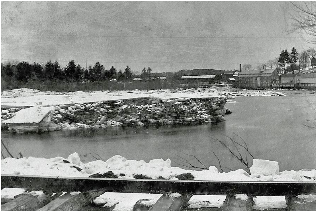
View of the damage along the Merrimack River facing the Commercial Street mills
