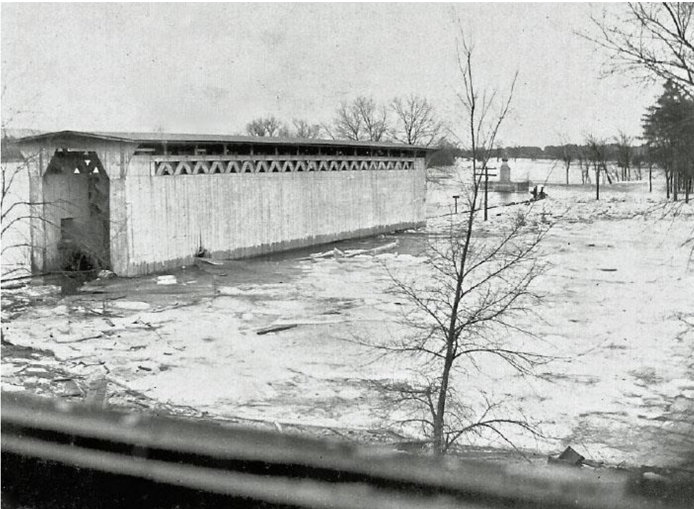
Close-up view of the Hannah Dustin Island Bridge (note the large chunk of ice sticking into the bridge wall)
