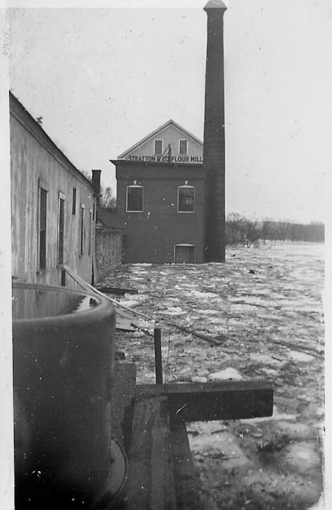
Back of Harris mill boiler across and Stratton's mill
