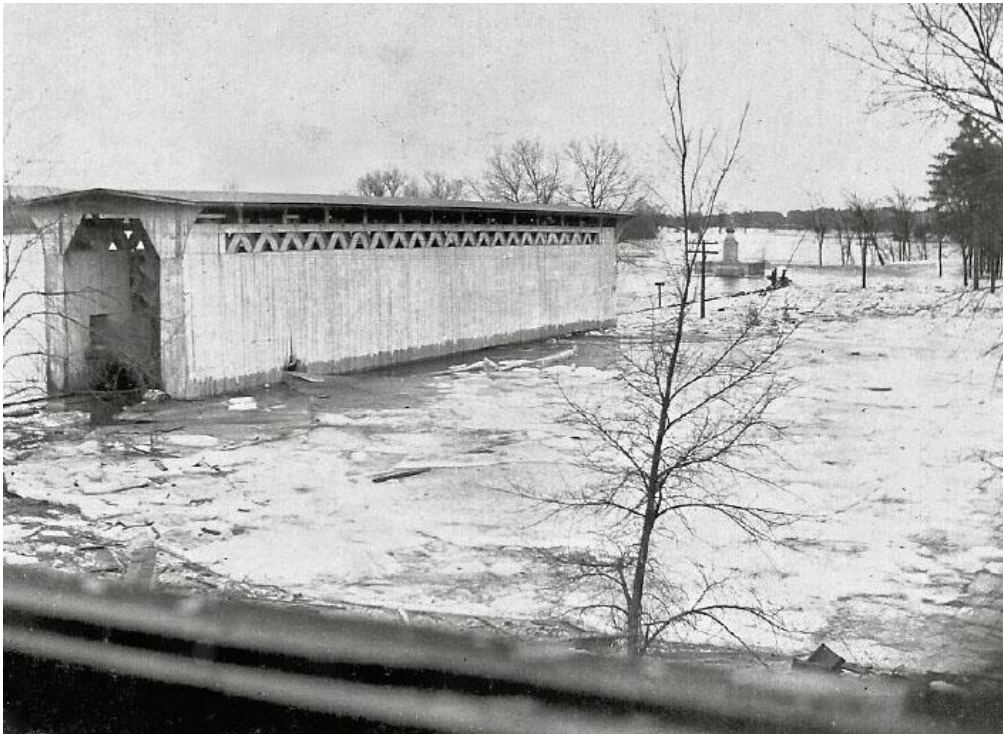
Close-up view of the Hannah Dustin Island Bridge (note the large chunk of ice sticking into the bridge wall)
