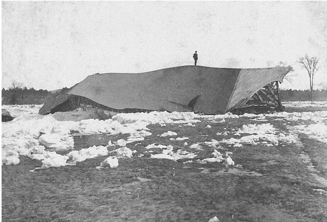
Boscawen-Concord Bridge resting on the interval after the flood
