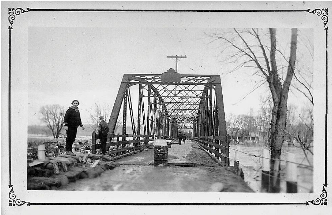
Boscawen-Canterbury Bridge over Merrimack River
