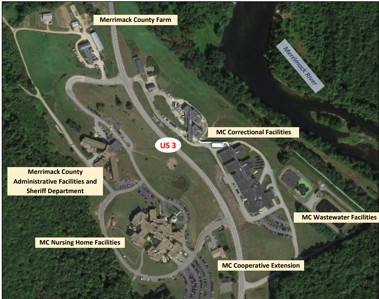
Figure 21 Merrimack County Facilities in Boscawen (US Route 3)
