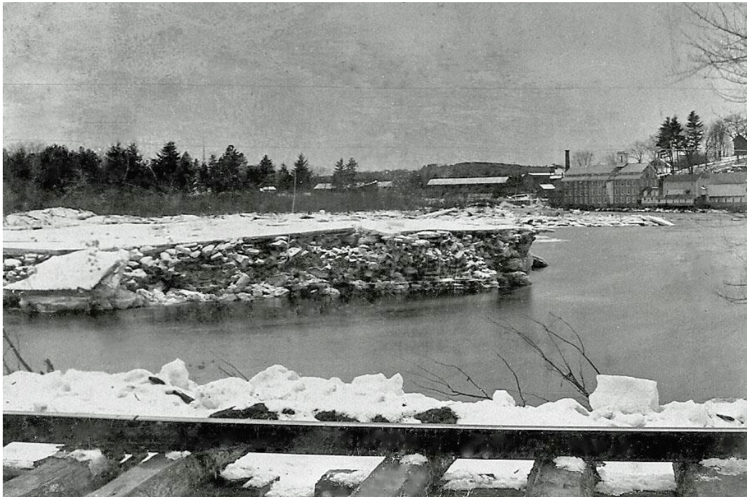
View of the damage along the Merrimack River facing the Commercial Street mills
