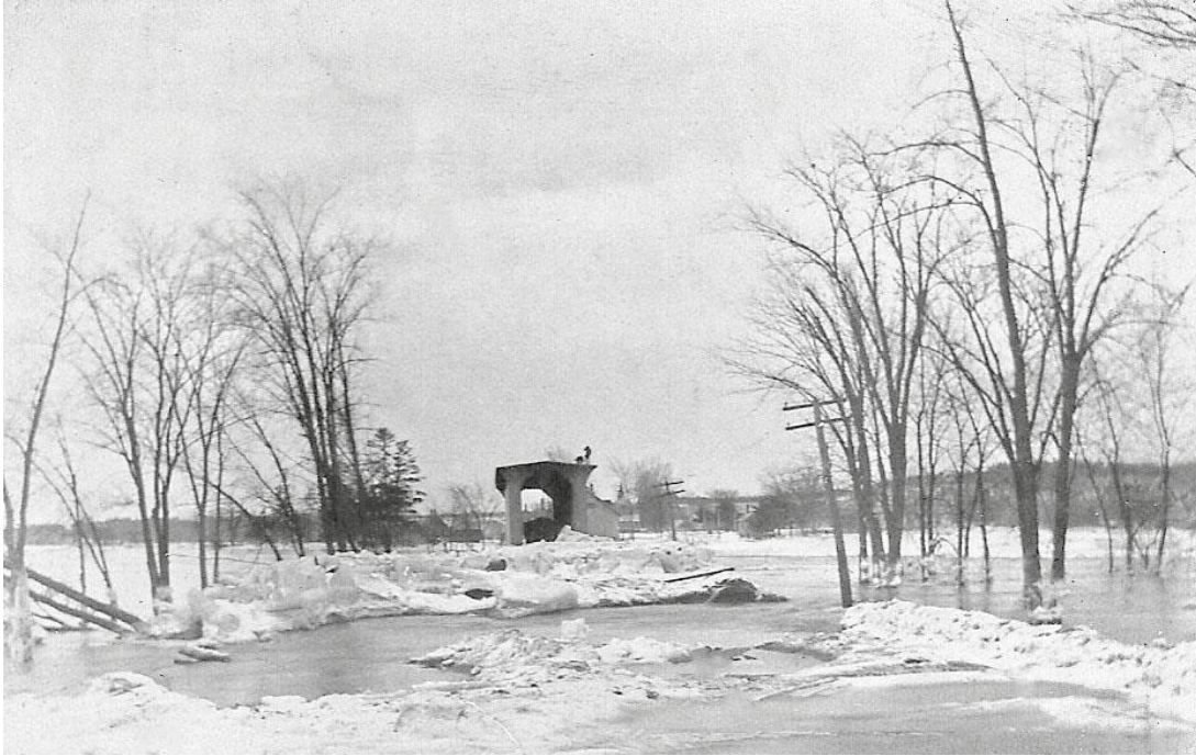
View of the Hannah Dustin Island Bridge completely under water
