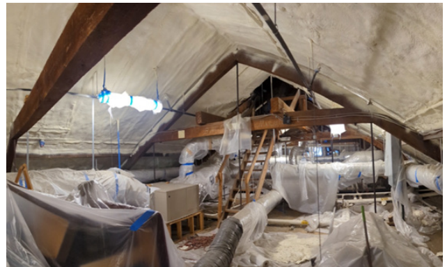
Pictured above - attic after spray foam is added
